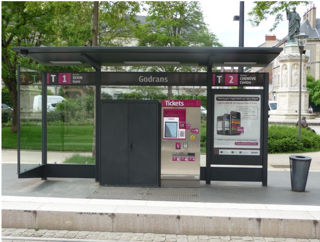
Equipements de station
